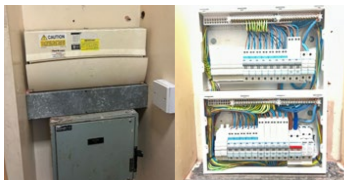
Before and after photos of a new fuseboard at one of our Schemes
