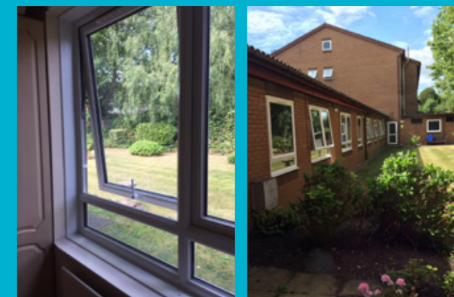
New double glazed UPVC windows at Young Court
